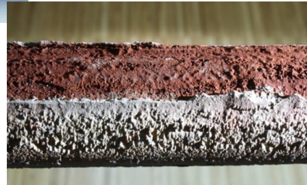
Economiser-tube - Low temperature corrosion
