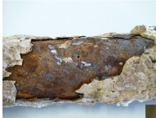
Superheater tube - High temperature corrosion
